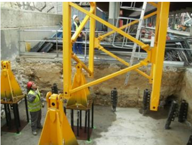
Figure 49. Erecting crane on platform 8.
