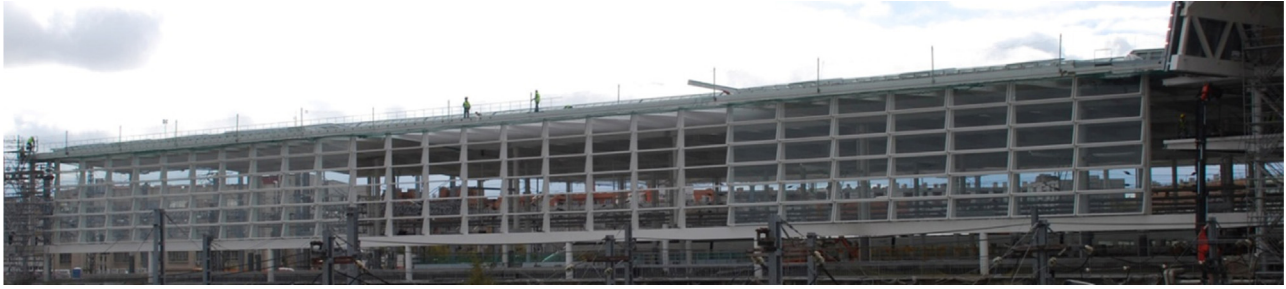
Figure 15. Curtain wall during construction.
