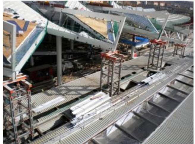
Figure 54. Shoring towers on platform 7.
