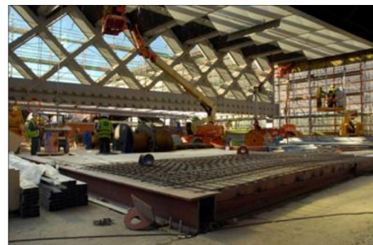
Figure 20. Construction of the steel grid prior to casting the concrete for the composite slab.
