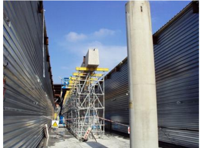
Figure 42. Demolition of canopies between provisional track protection tunnels.
