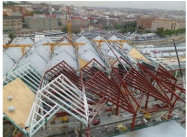
Figure 51. Bridge cranes over the high-rise canopies.
