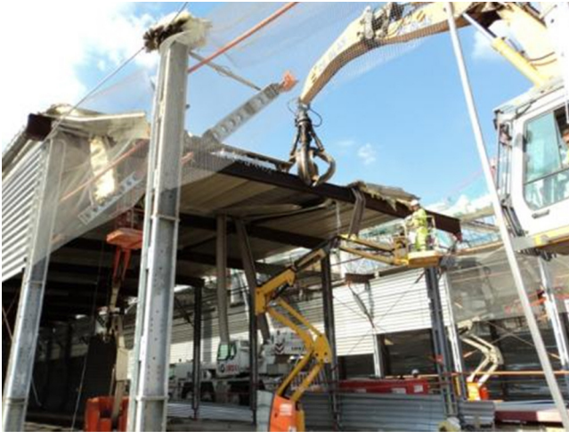
Figure 44. Demolition of provisional tunnels.
