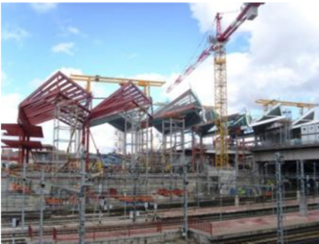
Figure 53. Shoring towers in the local train area.
