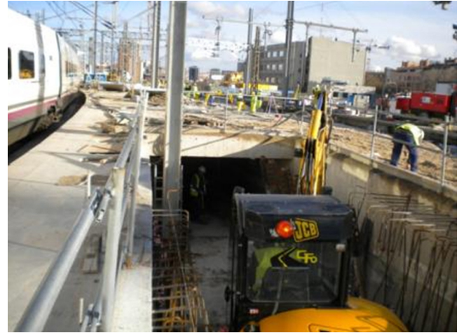
Figure 9. Catering ramps while under construction.
