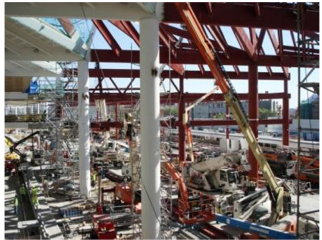
Figure 47. Coordination of machinery traffic.
