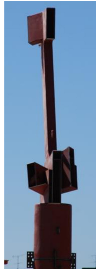
Figure 18. High-rise canopy node during assembly.
