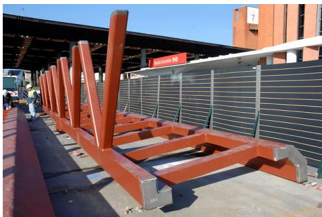
Figure 58. Roof module on the worksite.
