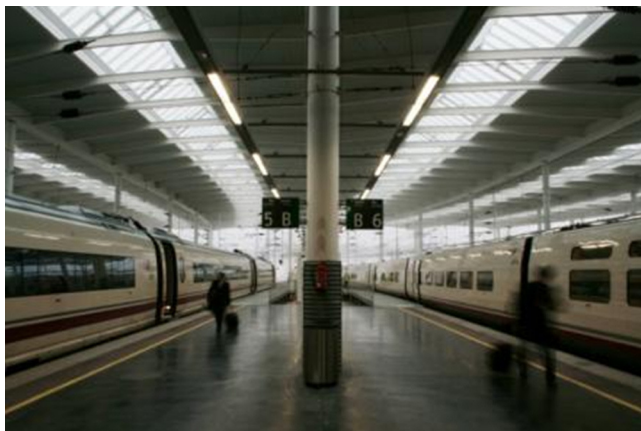
Figure 56. Finished low-rise canopies.
