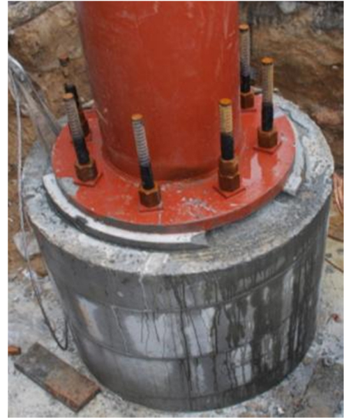
Figure 16. North side low-rise canopy foundations.
