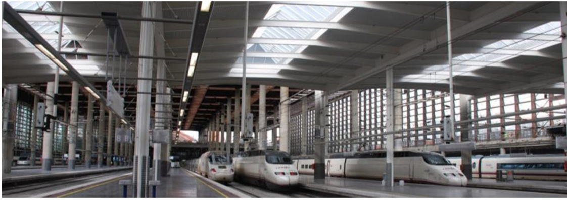
Figure 4. North side low-rise canopies.
