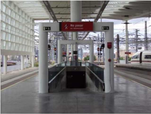
Figure 10. Finished catering ramps.
