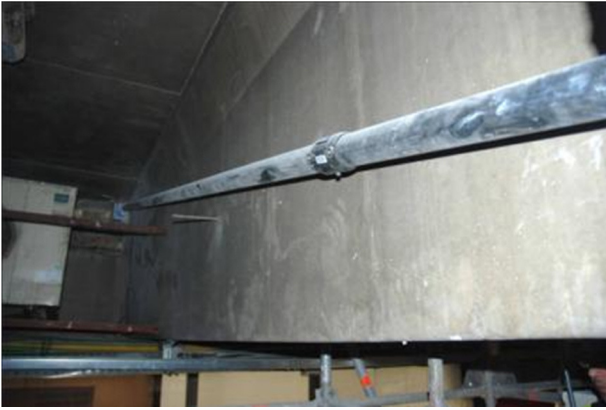
Figure 24. Existing beam strengthened with external post-tensioning.
