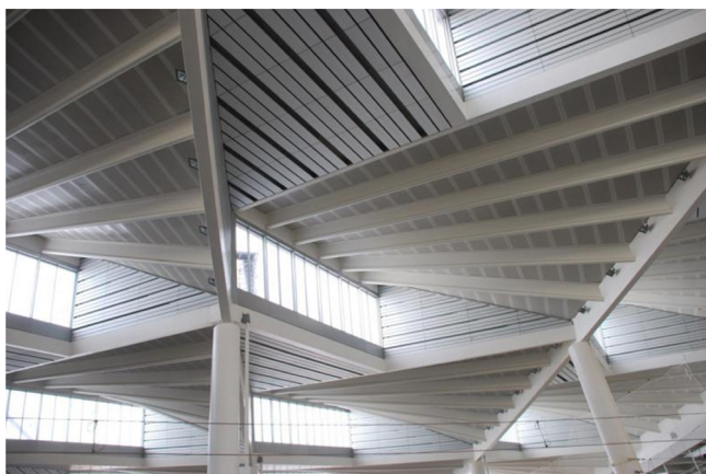
Figure 3. Indoor view of the finished high-rise canopy.
