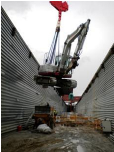
Figure 45. Platform access for machinery.
