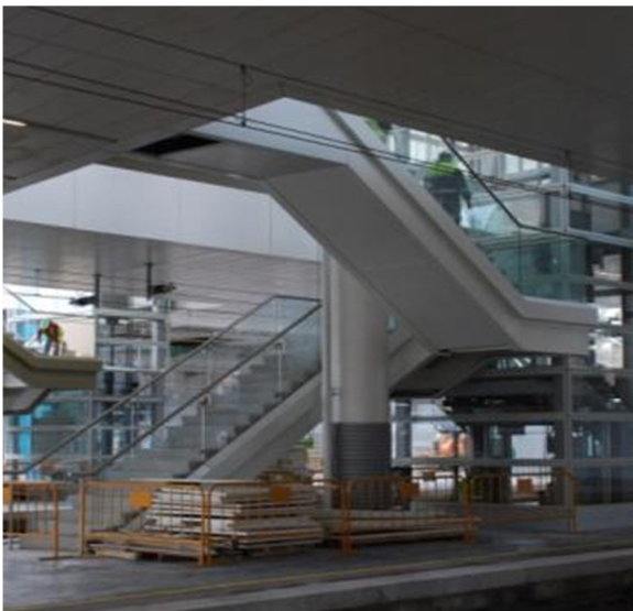
Figure 6. Stairway from platform to footbridge.
