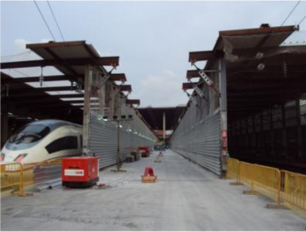
Figure 36. Provisional tunnels to protect tracks.
