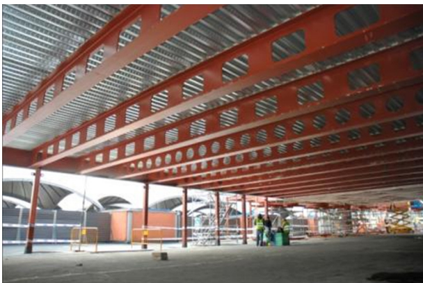
Figure 29. Composite beams with circular openings and “racecourses”.
