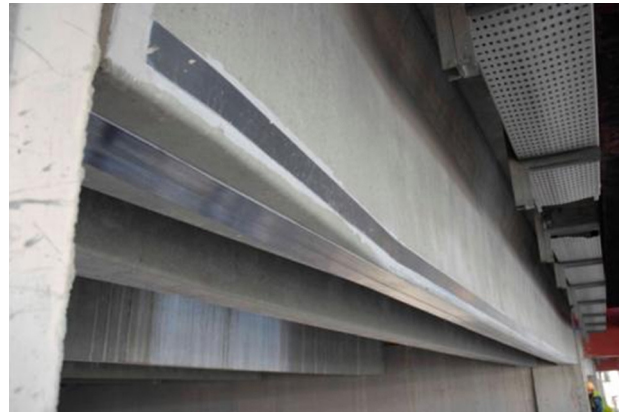
Figure 22. Carbon fibre flexural strengthening for secondary beams.
