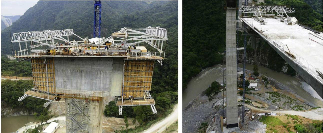
Figure 28. Overview of travelling formwork.
