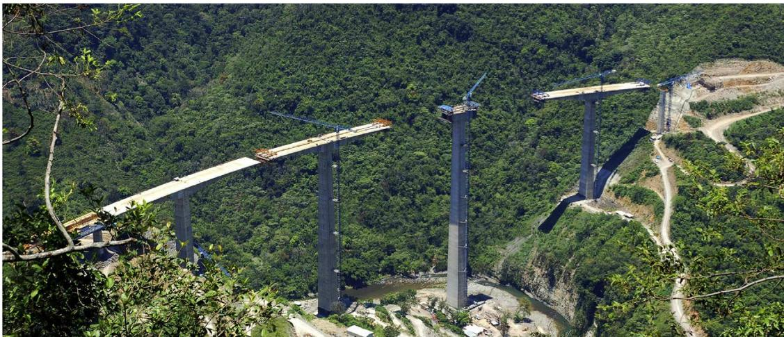
Figure 29. Simultaneous operation of three pairs of travellers.
