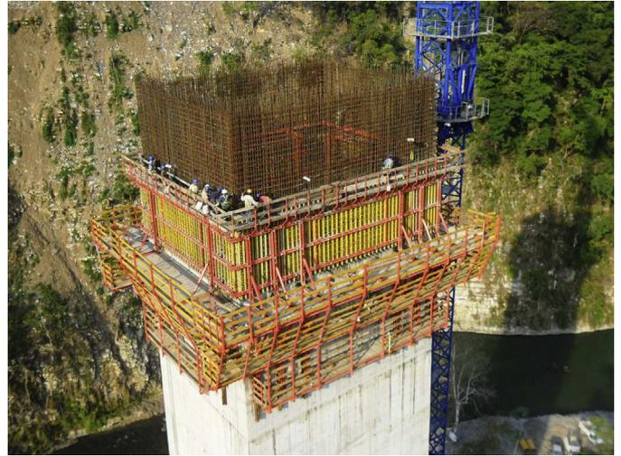
Figure 26. Self-climbing formwork on pier 4.
