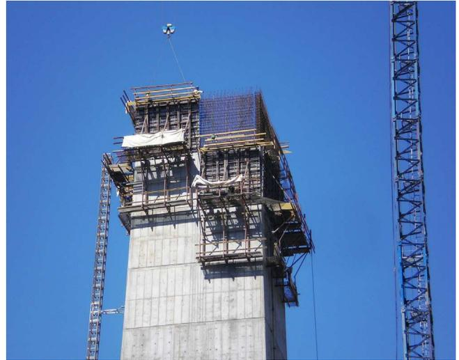
Figure 25. Conventional climbing formwork on piers 2, 3 and 5.
