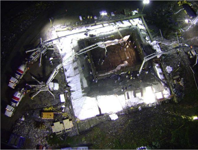
Figure 23. Continuous casting of pier 4 pile cap.
