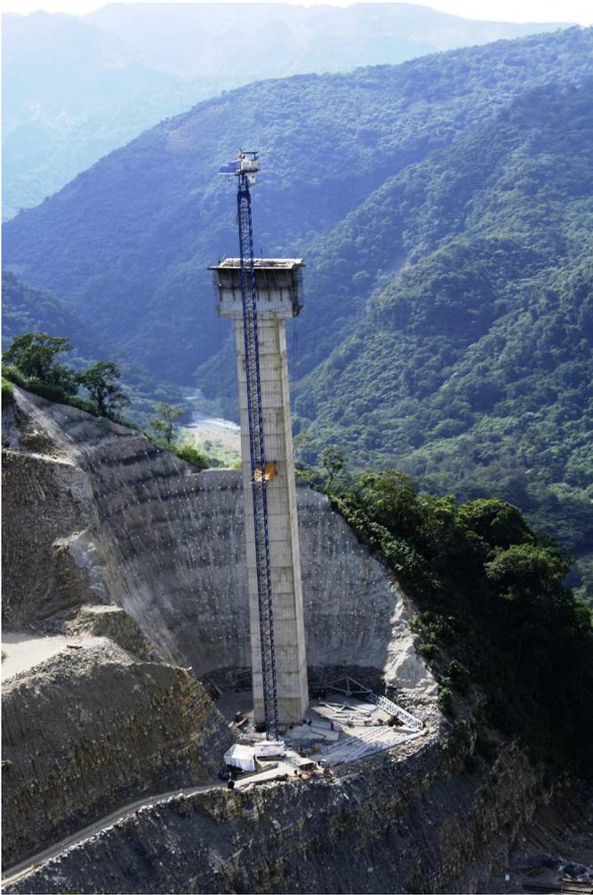
Figure 21. Pier 2 excavation.
