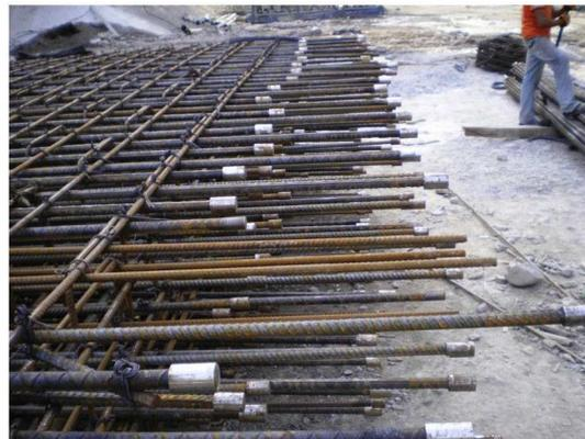
Figure 24. Pre-assembly of pier reinforcement.
