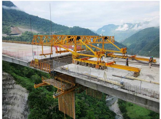
Figure 30. Locking a centre span.
