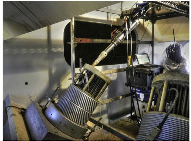
Figura 3. Isotension® Freyssinet.
