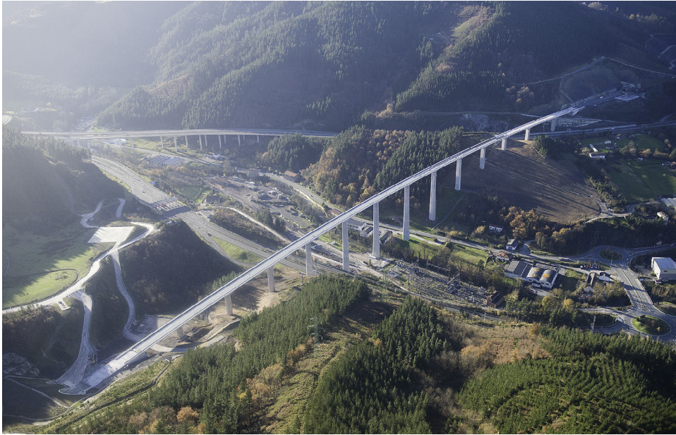
Figure 1. Finished River Deba Viaduct.
