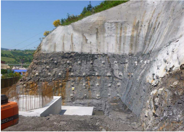
Figure 17. P-10 excavation with soil anchor pins and shotcreted banks.
