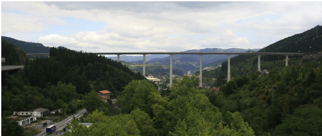
Figure 11. View of finished prestressed concrete viaduct.
