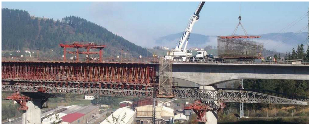
Figure 29. Positioning pre-assembled reinforcement on deck.
