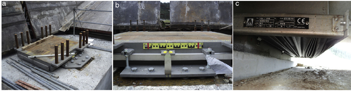
Figure 13. Bearing, ruler-based measuring system and dust cover.
