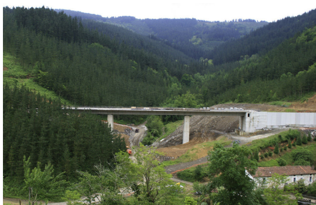
Figure 4. Olzaileko Brook Viaduct.
