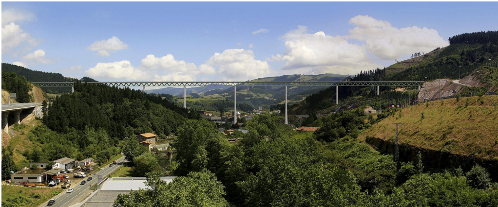
Figure 6. Simulation of composite truss solution with vertical piers chosen by ETS on the grounds of the typology study.
