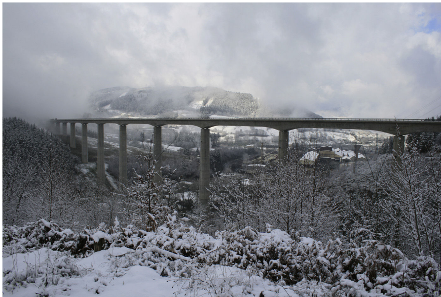
Figure 43. Viaduct during load test with lorries (4 February 2015).
