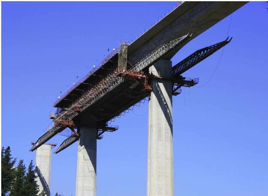
Figure 32. MSS support rings at top of pier.
