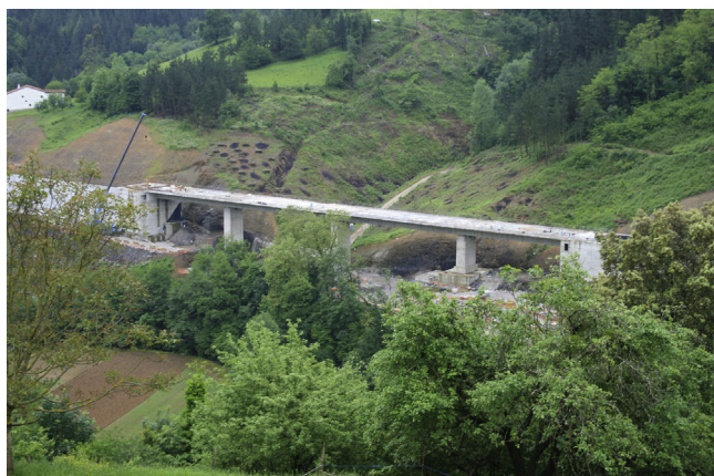
Figure 3. Altzeta Brook Viaduct.
