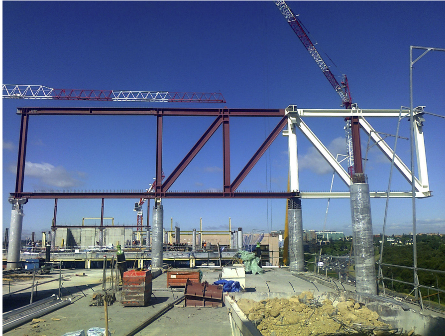
Figure 32. Assembly of trusses on composite columns.
