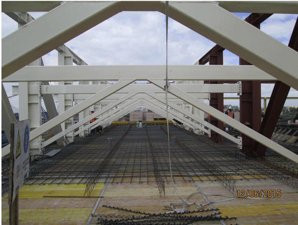
Figure 25. Supporting frames integrated into the roof structure.
