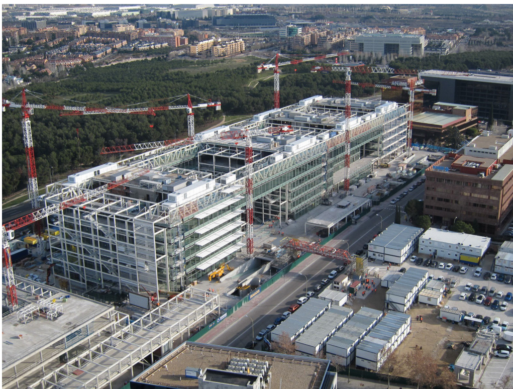
Figure 39. State of the project with the completed structure.
