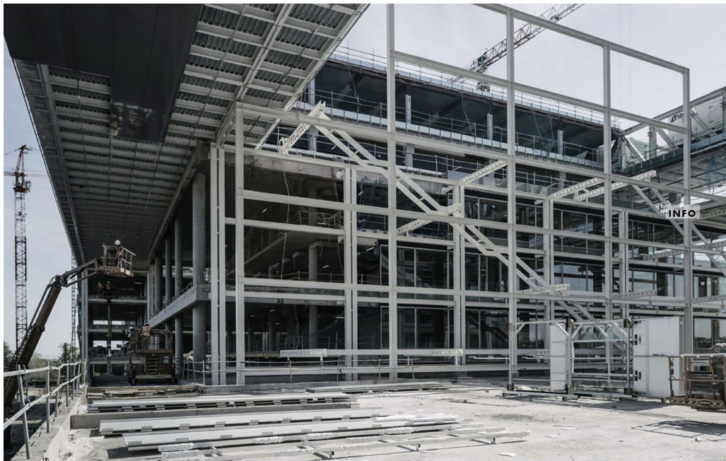
Figure 21. External steel structure and fire escape.
