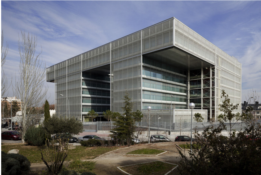
Figure 3. New Data Processing Centre building at calle Abelianas (stage I) [4].
