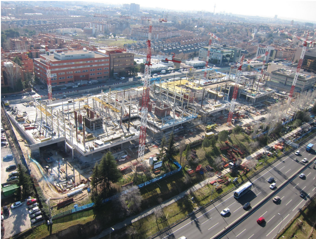
Figure 16. Execution of the structure above the ground level slab.
