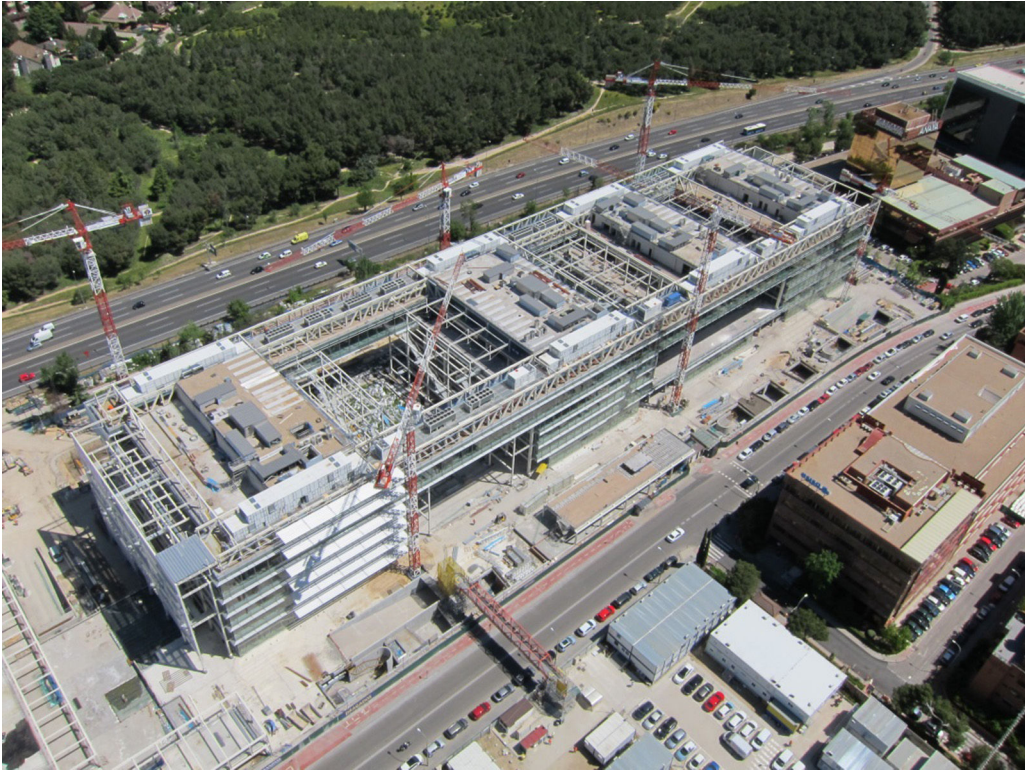
Figure 9. Bird's eye view of the roof (May 2016).
