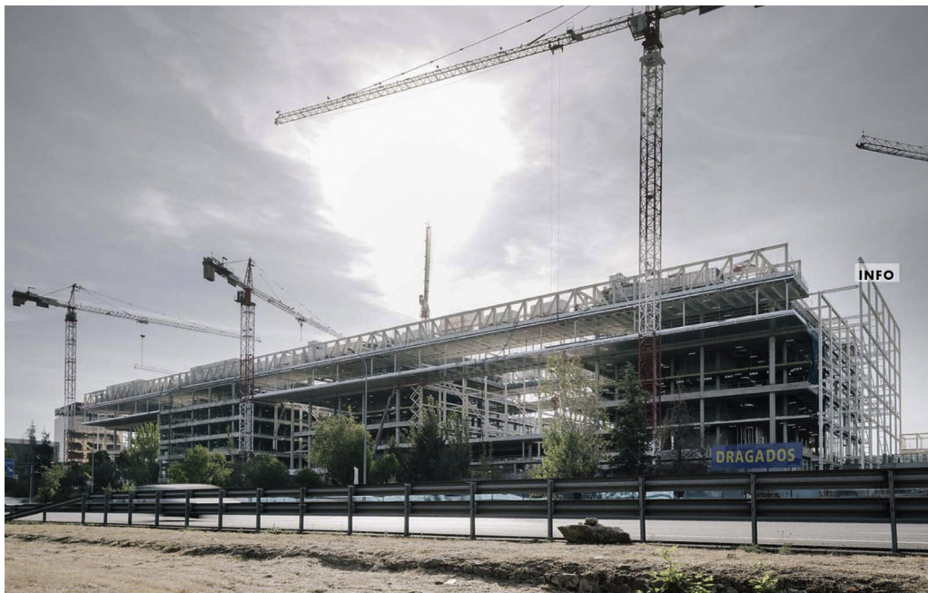
Figure 24. View of the trusses on the north façade.
