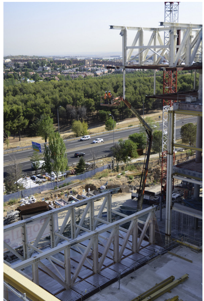
Figure 33. North bridge pre-assembled, awaiting hoisting.
