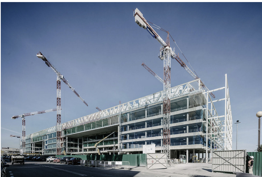
Figure 37. Figure of the project with the completed structure.
