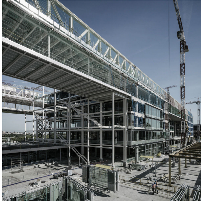
Figure 29. Figure of the roof structure and area between blocks.
