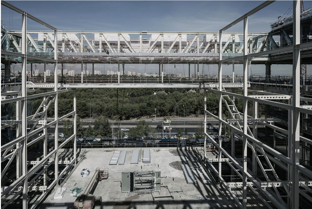
Figure 36. Figure of the structure of the finished “north bridge”.
