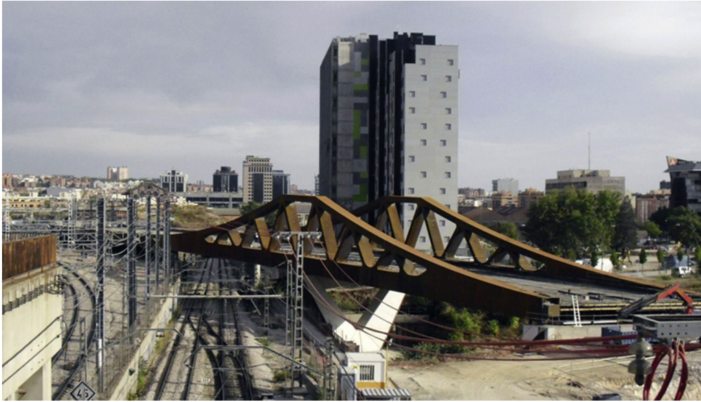
Figure 27. Web truss viaduct. Railway connection over calle Comercio. MC2 Ingeniería (2010).
