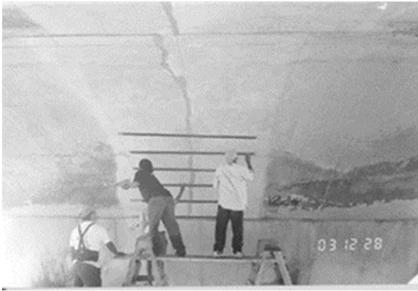
Figure 4. Rehabilitation of one of the cracked arches.
