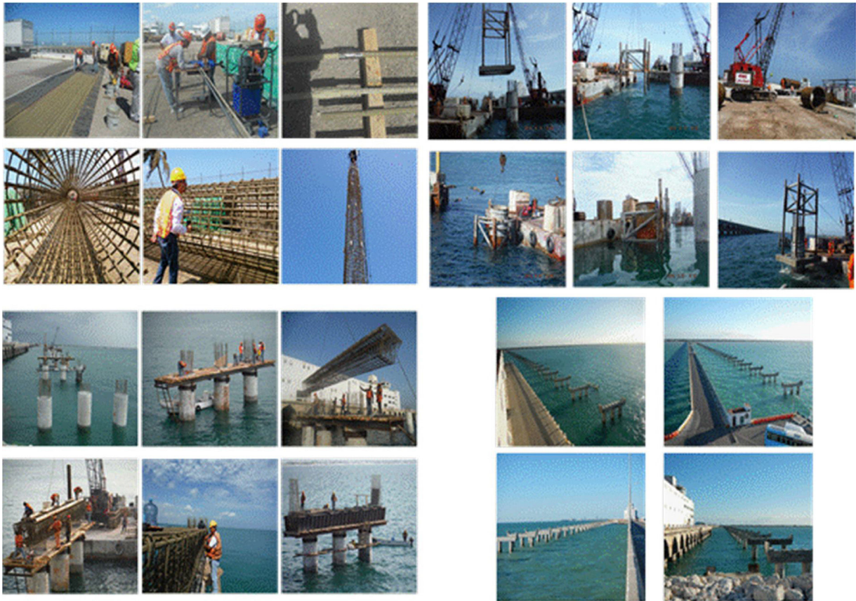
Figure 8. Construction process photographs: substructure construction stage.
