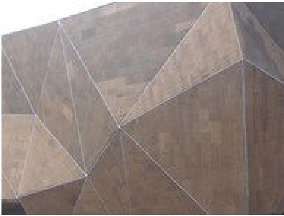
Fig. 1. External insulation of the Portugal Pavilion in Expo Shanghai 2010 with ICB.
