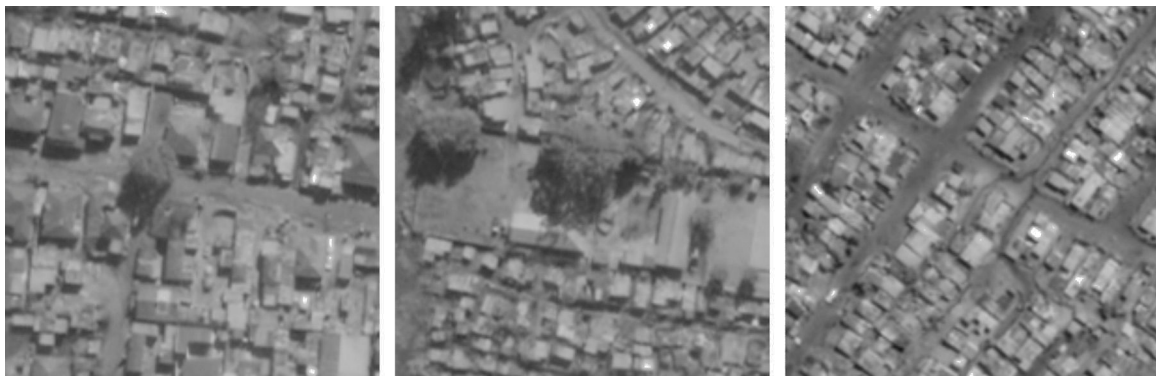
Fig. 4. Informal squatters (IS type1): the structure of the informal squatters is not stable. The dwellings of this category are shack type (made out of cardboard, wood, tin, etc.). Typically characterized by high building densities.
