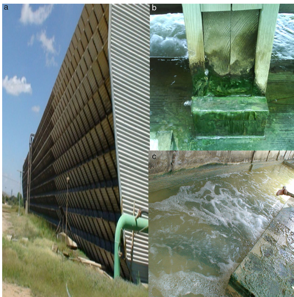
Figure 1. The cooling tower in the thermoelectric power plant of Villa de Reyes, San Luis Potosí, Central Mexico (a). The samples of biofilms composed by microalgae were taken at the top of the tower (b). Floor of the cancels in the top of the tower with microalgal mats, showing the turbulence of the water (c).
